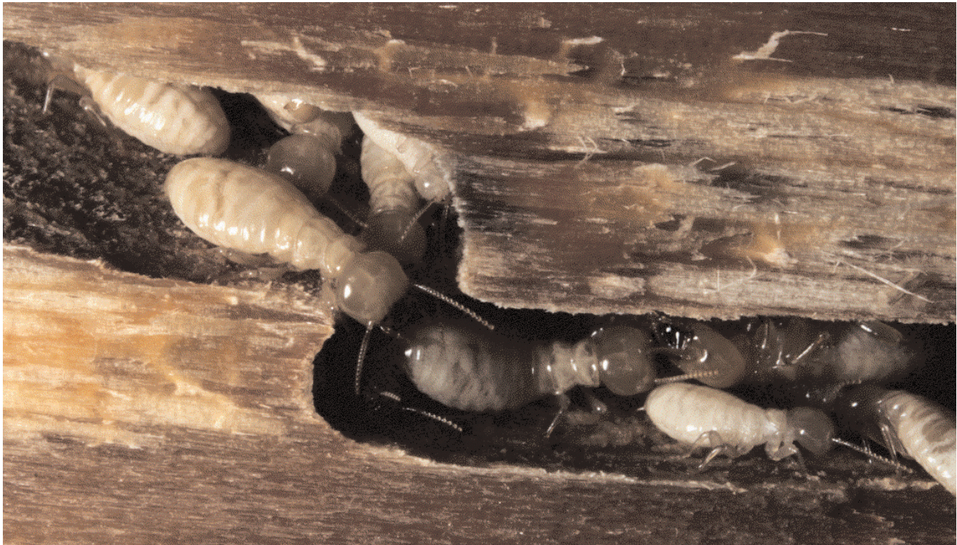
Termites damage your home by eating the soft grain of wood, leaving timbers with layered tunnels inside a thin shell.
